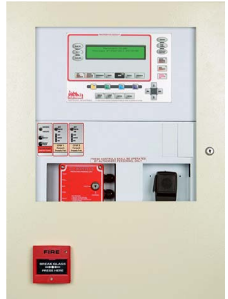
F120A Control Panel
